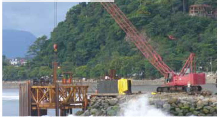
Marina breakwater, Costa Rica
