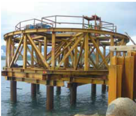
1. Installation of template
