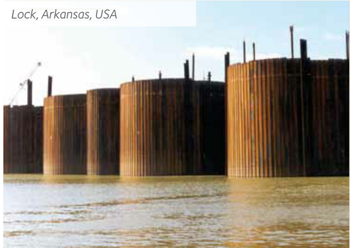
Diaphragm cells with 120^\circ junction piles.
